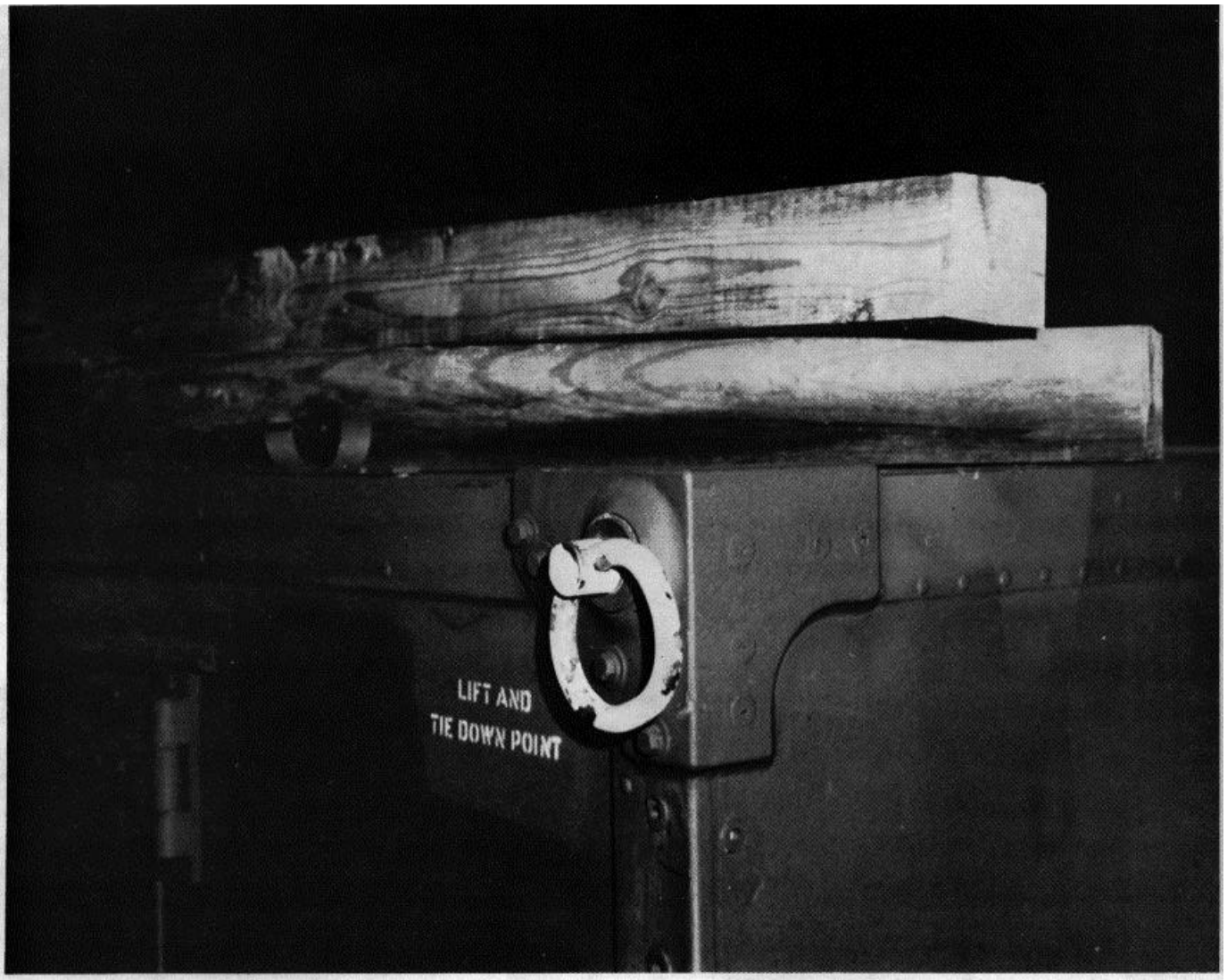
Figure 5. Location of rivets on vertical structural members.
