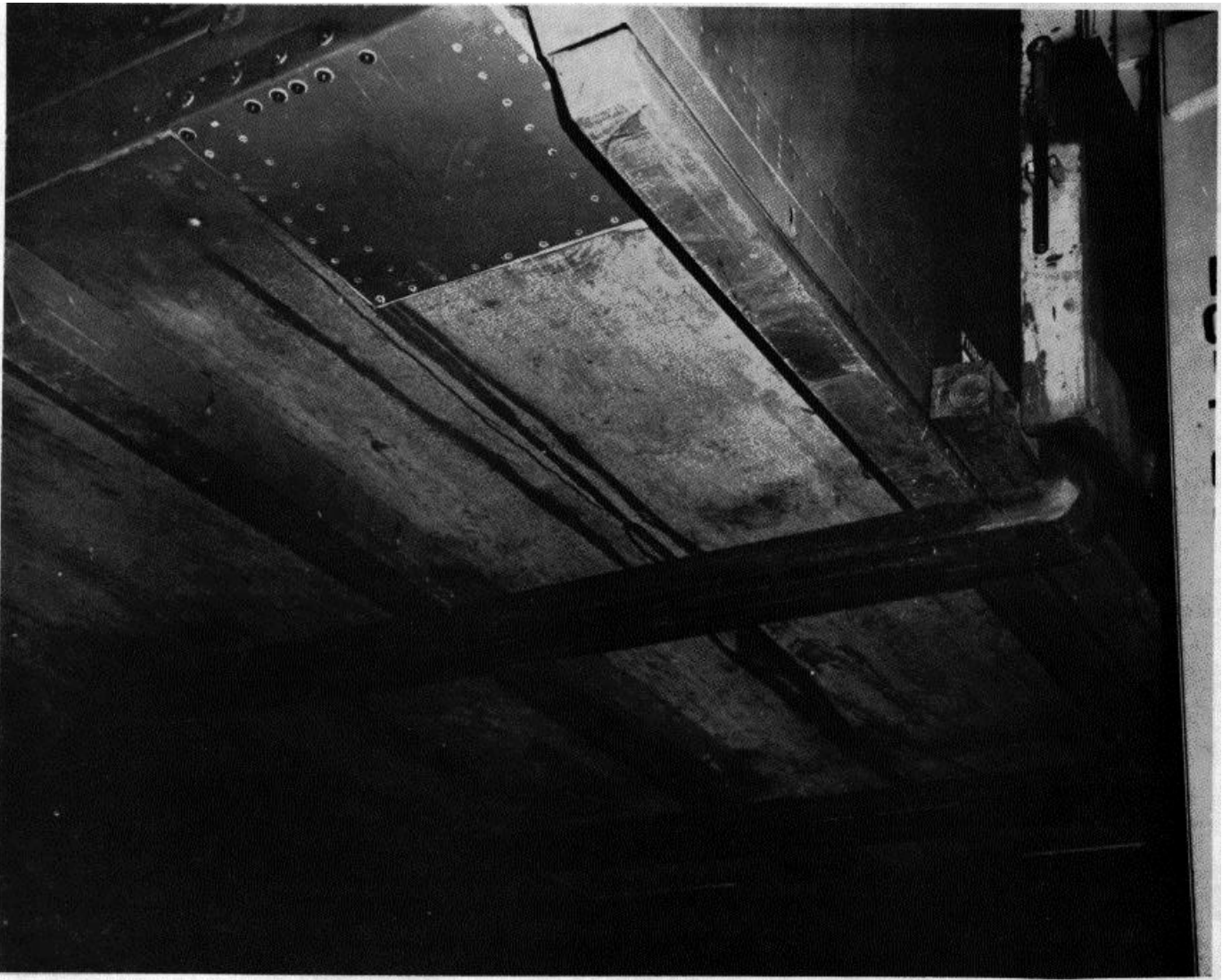
Figure 1. Forks/fork extensions reaching completely across the width of the shelter.
