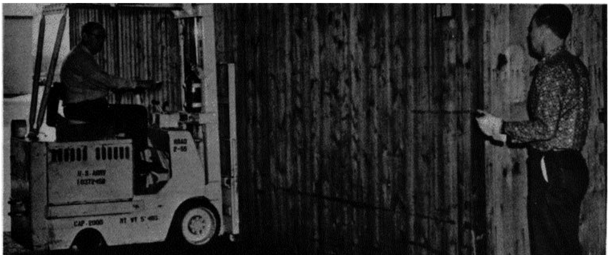
Figure 8. Using a single forklift truck to deposit elongated item following the step shown in figure 7.
